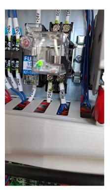
6. PLC input : Blue wire : DI-3-2( Robot E Stop input to PLC ), Module 3 and digital input 2
